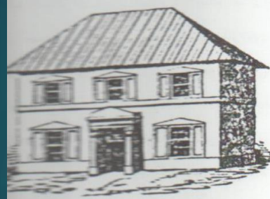
SOUTH AUSTRALIAN BANK.
